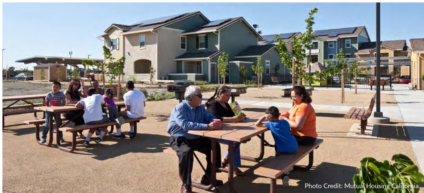
Zero net energy affordable housing project for farmworker families in Woodland, CA.
