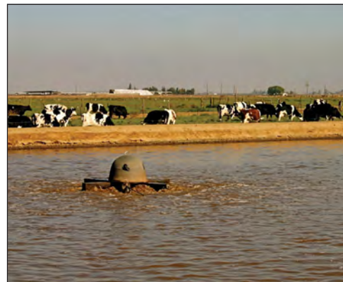
Aeration of manure lagoons with Circul8 Systems
