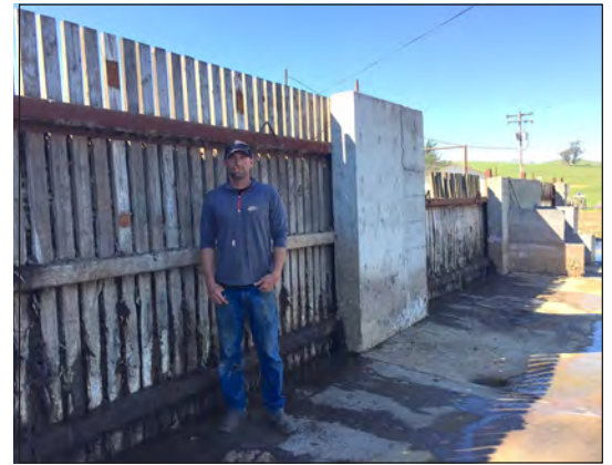
Weeping wall solid separator
