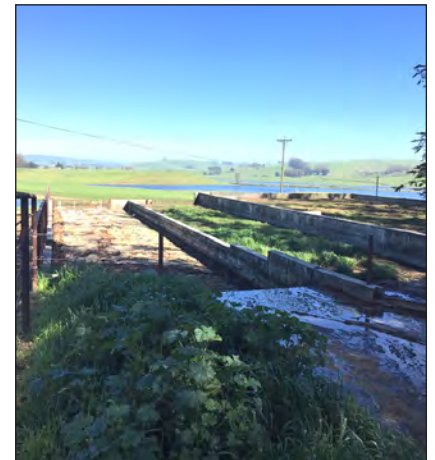
Gravity-fed channels from barn to three flush pits
